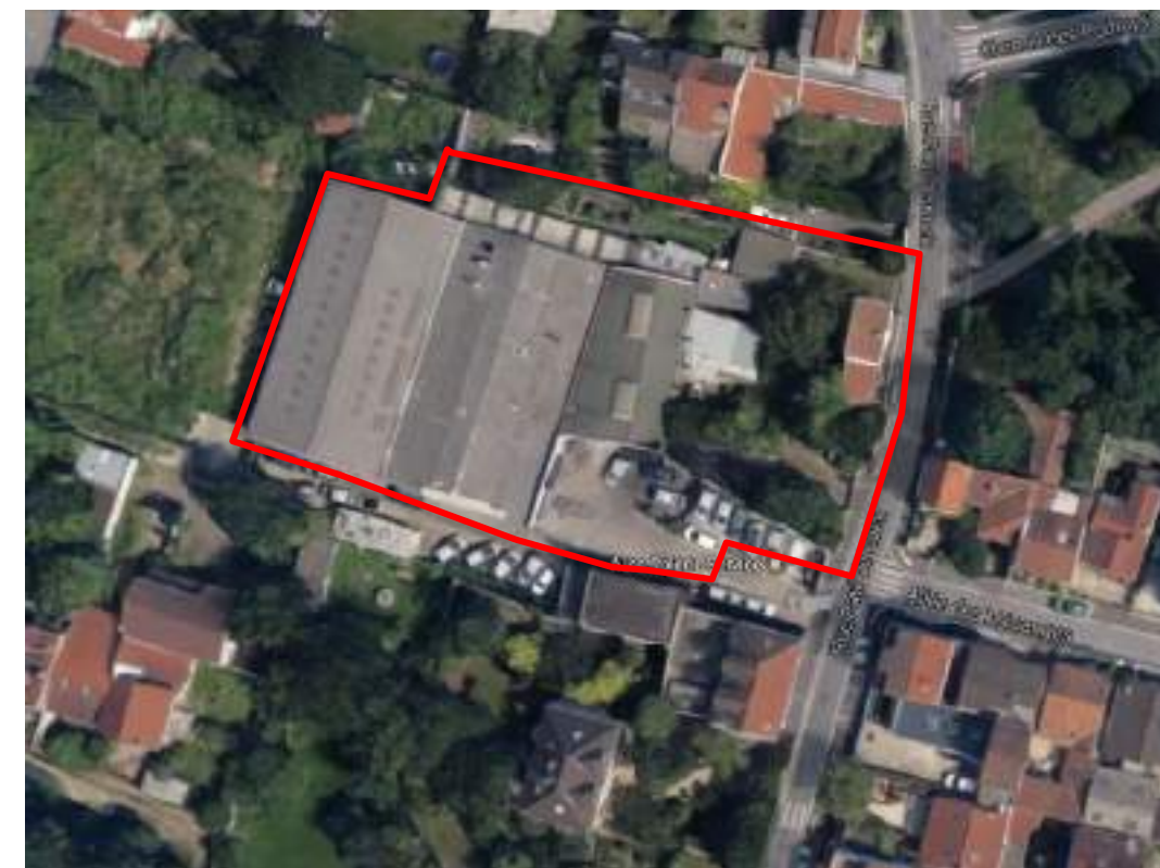
Figure 131: Localisation du garage ATS - source: Google maps
